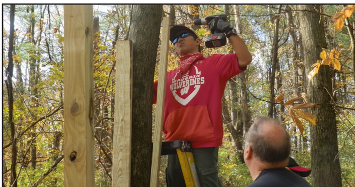
Construction of exclosure.
